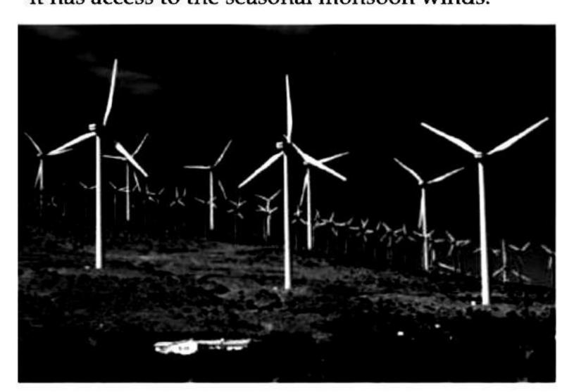
The electrical generators used on wind turbines in sites like Muppandal, produce an output AC of 240 V and a frequency of 50 Hz even when the wind speed is fluctuating. A transformer may be required to increase or decrease the voltage so it is compatible with the end usage, distribution or
